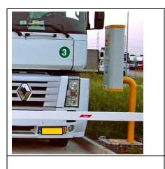
Ticket printer and information machine – placed at the barrier, easy to handle, can be accessed from a truck as well (elevated)
